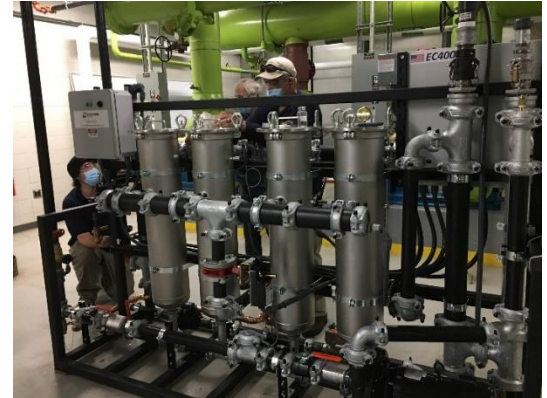
ElectroCell EC4000 installation
