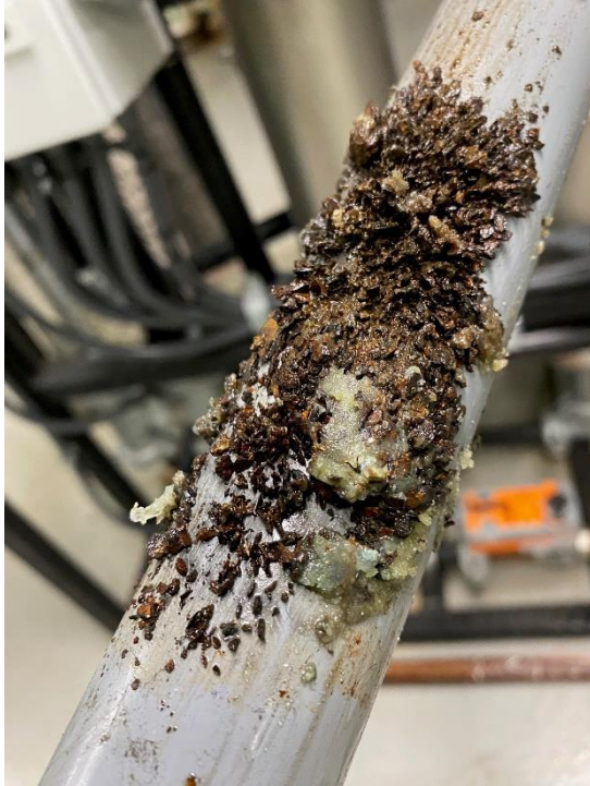
Rust removed from circulating water in condenser water system by magnet.
