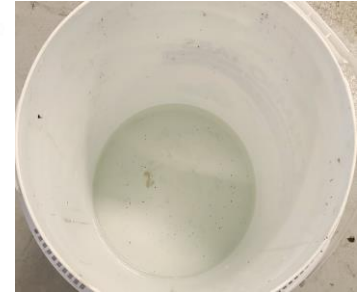
Condenser water before start-up Particles > 25 micron,
