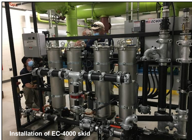
Cleaning of ElectroCell skid
