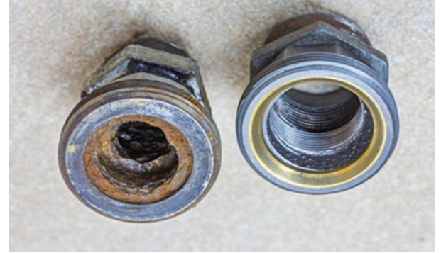
Corrosion removed on inside of piping reducing friction.
