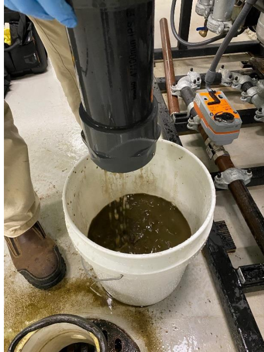
Dissolved solids removed from cleaning of static mixers.
